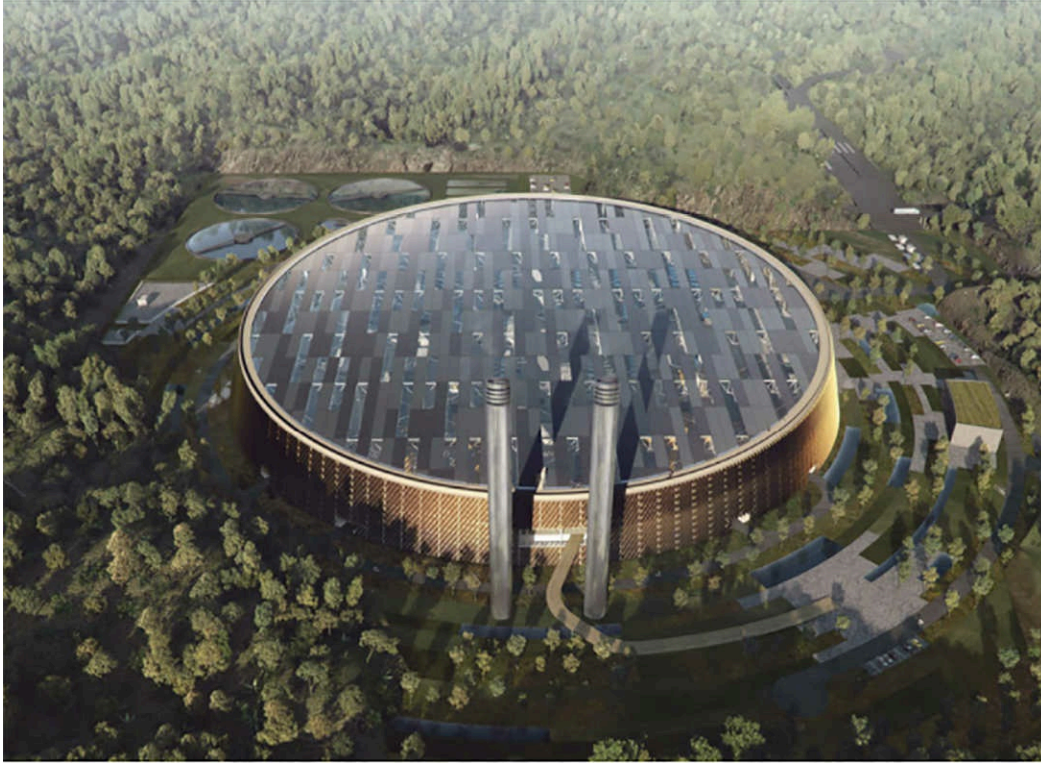
Figure 69. China has recently built the world's largest waste-to-energy plant in Shenzhen. It will burn more than 5,000 tons of waste per day, producing 168 megawatts of electricity. The roof is covered with 44,000 square meters (474,000 square feet) of solar panels. The visitors center will focus on education in waste management and recycling. 195
